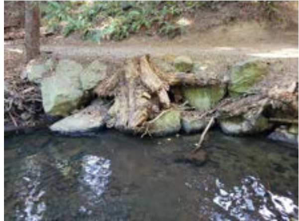
Photos 49 & 50. LWD structure along right bank at km 1+030 beginning to rot – soil could be used to backfill bank behind structure to further anchor it into bank (above left; Aug. 25, 2021). LWD structure holding up right bank and above low water level at km 1+037 – could install additional LWD structures closer to low water mark (above right; Aug. 25, 2021).
