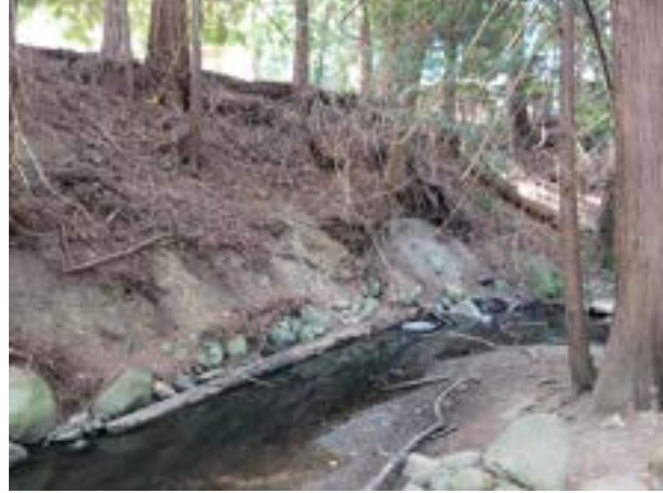
Photos 53 & 54. Steep ravine bank along right bank of stream between approximately km 1+037 and 1+052 that could use terraces and planting to stabilize slope and provide cover/shade to stream (above left; Aug. 25, 2021). Steep right bank at km 1+105 that could use terraces and planting to stabilize slope and provide cover/shade to stream (above right; Aug. 25, 2021).
