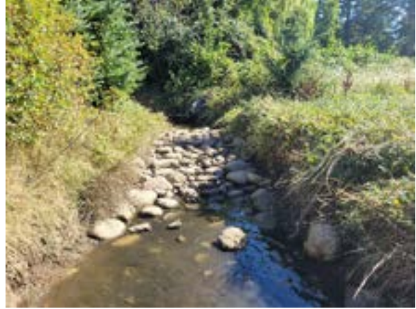
Photos 11 & 12. Upstream end of constructed side channel from mainstem (with invasive species), looking downstream toward side channel. Exposed cobbles at inlet of channel, no surface connectivity at time of site visit (above left; Aug. 12, 2021). Constructed riffle at downstream end of side channel, no scouring at toe of riffle (above right; Aug. 12, 2021).
