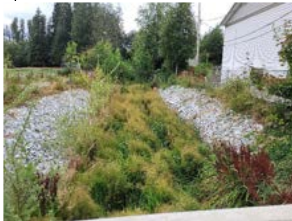
Photos 69. Planted riparian vegetation along left bank of Reach 4, immediately downstream of Noel Avenue channel in-filled with vegetation (above; Aug. 26, 2021).
