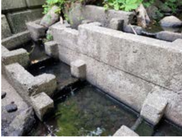
Photos 65 & 66. Constructed fish ladder upstream of Dogwood Avenue acting as low flow barrier to salmonids (above left; Aug. 26, 2021). Pedestrian bridge at km 1+970 in Reach 4; pedestrian path along right bank in this section of Reach 4 (above right; Aug. 26, 2021).
