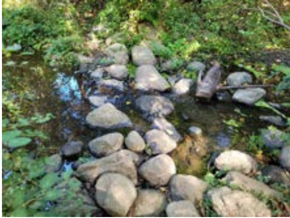
Photos 78 & 79. Constructed riffles in the Salish Park section of Reach 5 – both in good condition with no maintenance required (above left and right; Sept. 2, 2021).
