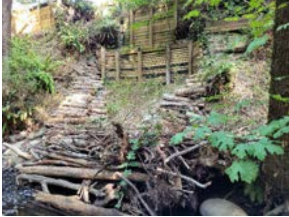
Photos 35 & 36. Retaining wall constructed by property owner along eroding left bank in HU G2-3 (above left; Aug. 20, 2021). Riprap armoured right bank preventing pedestrian path from eroding into stream in lower portion of Reach 3. Steep ravine bank to the west of the walking path. Recommend riparian planting between riprap wall and pedestrian path. Dense English ivy along left bank (above right; Aug. 25, 2021).
