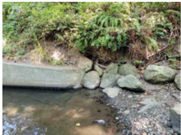
Photos 32 & 33. Fish ladder downstream of Balmoral Avenue potentially acting as fish barrier during low flows (above left; Aug. 20, 2021). Water flowing around left bank of fish ladder instead of all through centre of fish ladder downstream of Balmoral Avenue (above right; Aug. 20, 2021).
