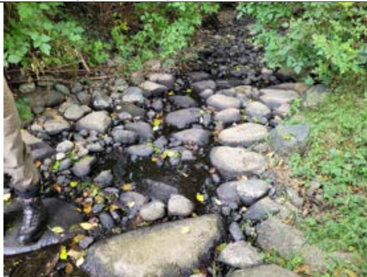
CR4.1 – looking downstream (Aug. 26, 2021)
