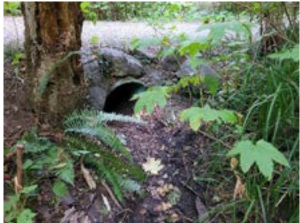
Photos 24 & 25. Spawning gravels along bank in HU P1-2 at km 0+385 (above left; Aug. 19, 2021). Culvert beneath walking path connecting wetted area to the west and Brooklyn Creek during high flow events (above right; Aug. 20, 2021).
