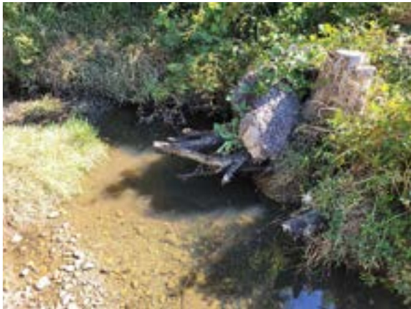
Photos 13 & 14. Installed LWD/boulder complex in pool upstream of constructed riffle in side channel; providing cover and habitat complexity for fish (above left; Aug. 12, 2021). Himalayan blackberry covering banks of side channel, looking upstream (above right; Aug. 12, 2021).
