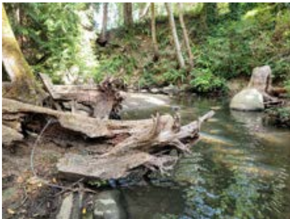
Photos 51 & 52. LWD structure along right bank at km 1+060 beginning to rot – could be supplemented with an additional stump or root wad (above left; Aug. 25, 2021). Rotting LWD structure along right bank in pool at km 1+290 – good candidate pool for larger LWD (above right; Aug. 25, 2021).
