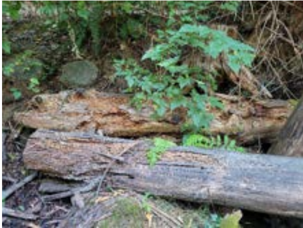
Photos 49 & 50. LWD structure along right bank at km 1+030 beginning to rot – soil could be used to backfill bank behind structure to further anchor it into bank (above left; Aug. 25, 2021). LWD structure holding up right bank and above low water level at km 1+037 – could install additional LWD structures closer to low water mark (above right; Aug. 25, 2021).
