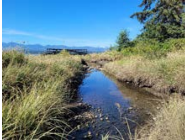
Photo 5. Eroding hardpan banks upstream of walking bridge, looking downstream toward estuary (above left; Aug. 12, 2021).
