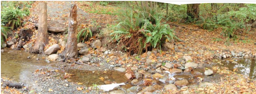
Photo 4. Temporary log bridge used at km 1+200 showing gravel reserved during bridge decommissioning for riffle construction. (Aug. 9 2010).
