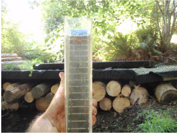
Photo 5. Turbidity measurement taken at temporary crossing during bridge construction. (Aug 9, 2010).
