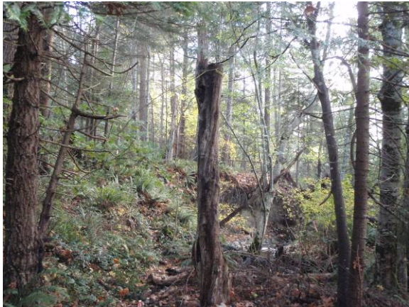
Photo 6. Wildlife tree installed during decommissioning of temporary tote road (Aug 9, 2010).
