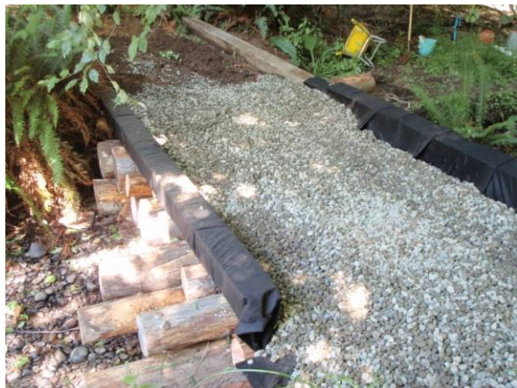
Photo 4. Temporary log bridge used at km 1+200 showing gravel reserved during bridge decommissioning for riffle construction. (Aug. 9 2010).
